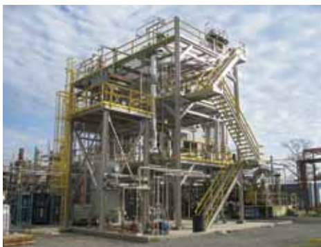
Gevo, the company that provided ATJ for an Air Force demonstration, commissioned a facility that can convert 10,000 gallons of isobutanol feedstock into approximately 8,000 gallons of bio-jet fuel.
